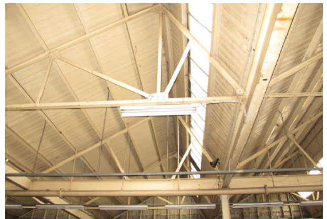
Figure 3.13 Detail of the 1914 steel roof framing system.
