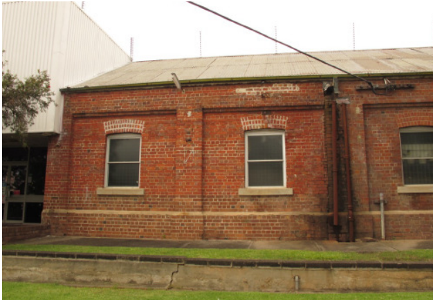
Figure 3.8 Detail of the arcaded brickwork adjacent the c1970 entry. Note the damage to the brickwork from the broken guttering and the inappropriate mortar repairs.
