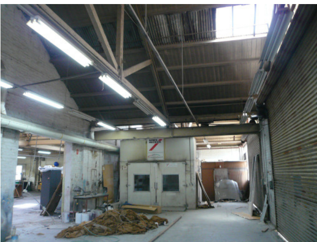
Figure 3.12 South eastern corner of the building, the 'indent' space resulting from the 1914 structure wrapping around an earlier building.
